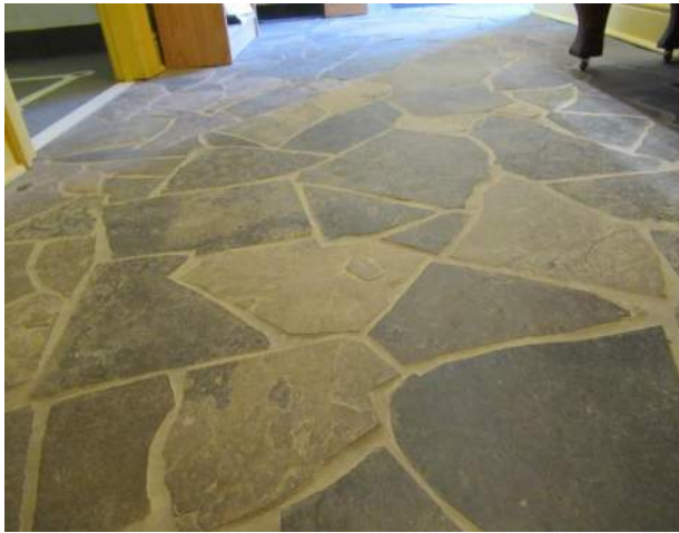
Picture INT 05 Components – Stone tile flooring Location – 2008 Addition
