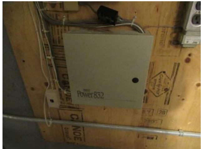
Picture ME 12 Components – DSC Security panel Location – Basement
